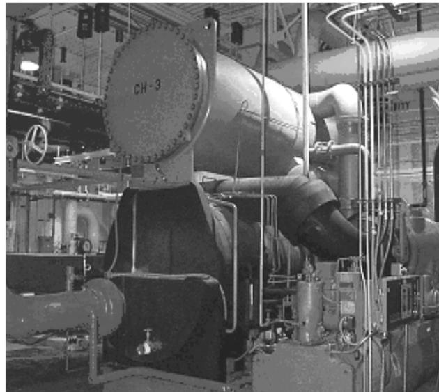
Chiller energy can account for 10 to 20% of total cleanroom energy use. The majority of annual chilled water use goes to medium temperature chilled water requirements – 55°F for sensible cooling and 60 to 70°F for process cooling loads. When outside air temperatures are cool and humidity is low (i.e., no low-temperature water is needed for dehumidification), 100% of the chilled water is for medium temperature loop uses.
